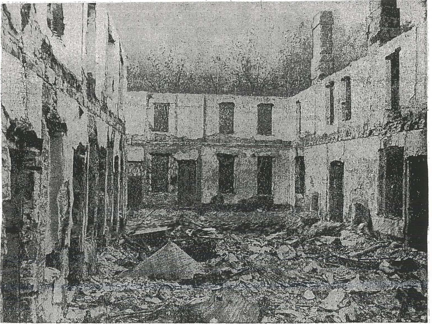
A southward view through the interior of the north-wing of the Tassajara Hot Springs Hotel after the fire of September 8, 1949. The main entrance is on the right, below and between the two chimneys. From the September 10, 1949 edition of the San Francisco Chronicle .
