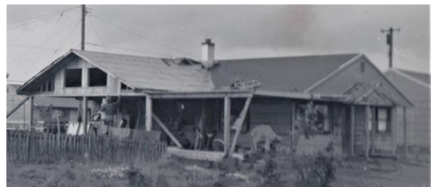
16 Adding carport, garage, and storm entrance, 1958
