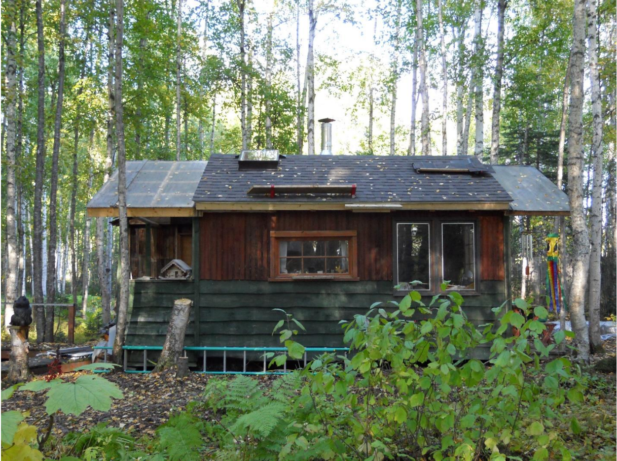
22 The Question Lake cabin with new roof and skylight in 2012
