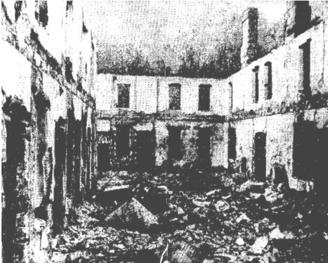
Guests and employees fought side by side in a fruitless effort to save this main building at Tassajara. But all that remains are arches, ambers and rubble, surrounded by thick walls and chimneys. Nine cabins and other buildings were also destroyed at the swank resort. There is enough food and water for the 50 guests and employees, however.
