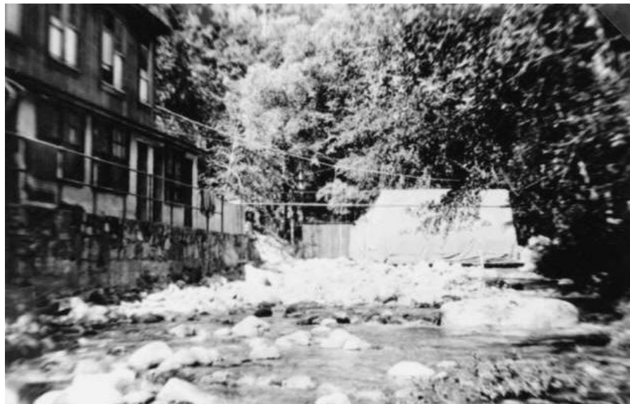
The wooden vapor bath and cooling tent. The wooden part was replaced by a concrete structure in 1928 or 1929.
