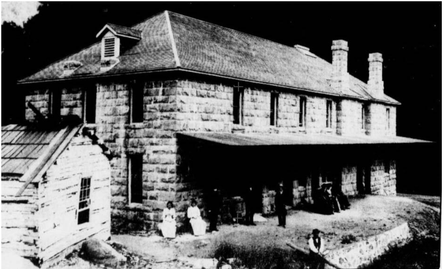
The Tassajara Hot Springs Hotel, as photographed on its completion in early July of 1893. The zendo, upper garden, the garden cabins and the library now occupy this site.
