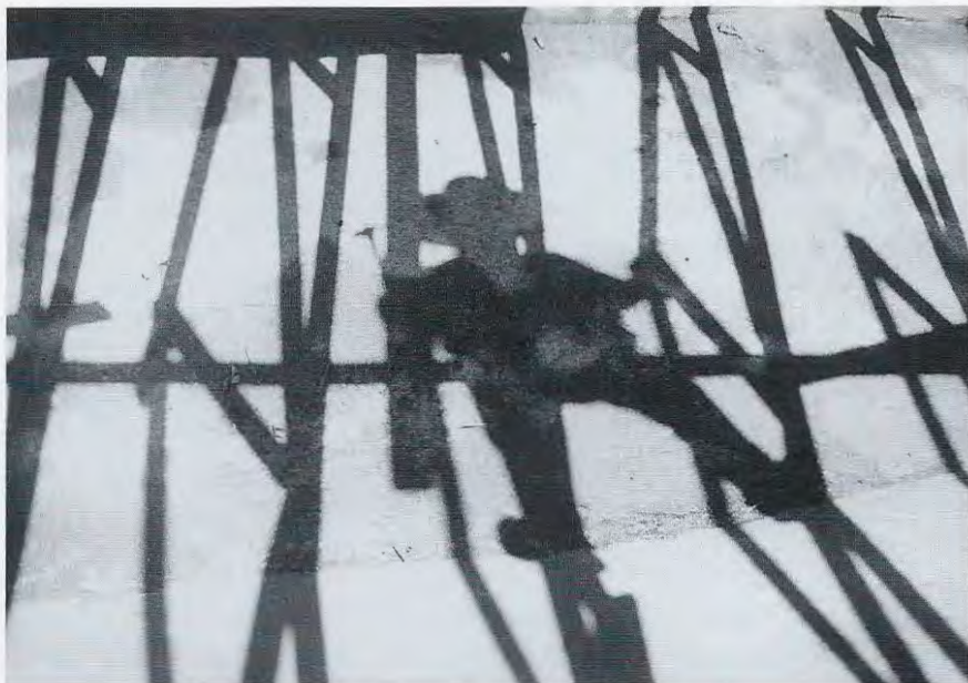
Rebuilding the roof of the water reservoir at Tassajara
