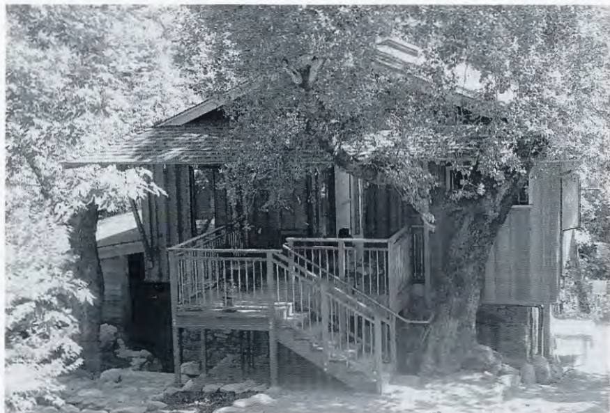
New entrance to the student dormitory above the new stone dining room
