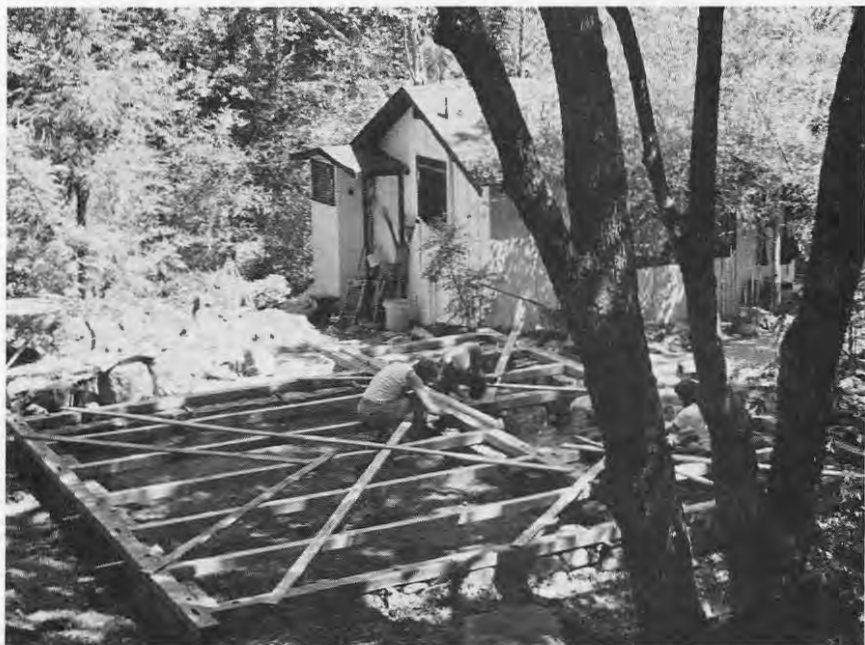
Building the Suzuki-roshi memorial cabin at Tassajara
