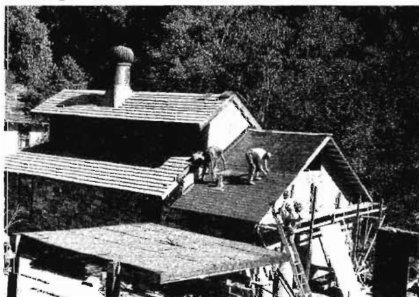
Roofing the kitchen
