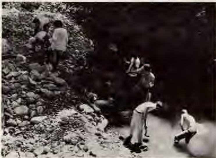
Students gathering and screening mortar gravel for the stone walls of the new kitchen
